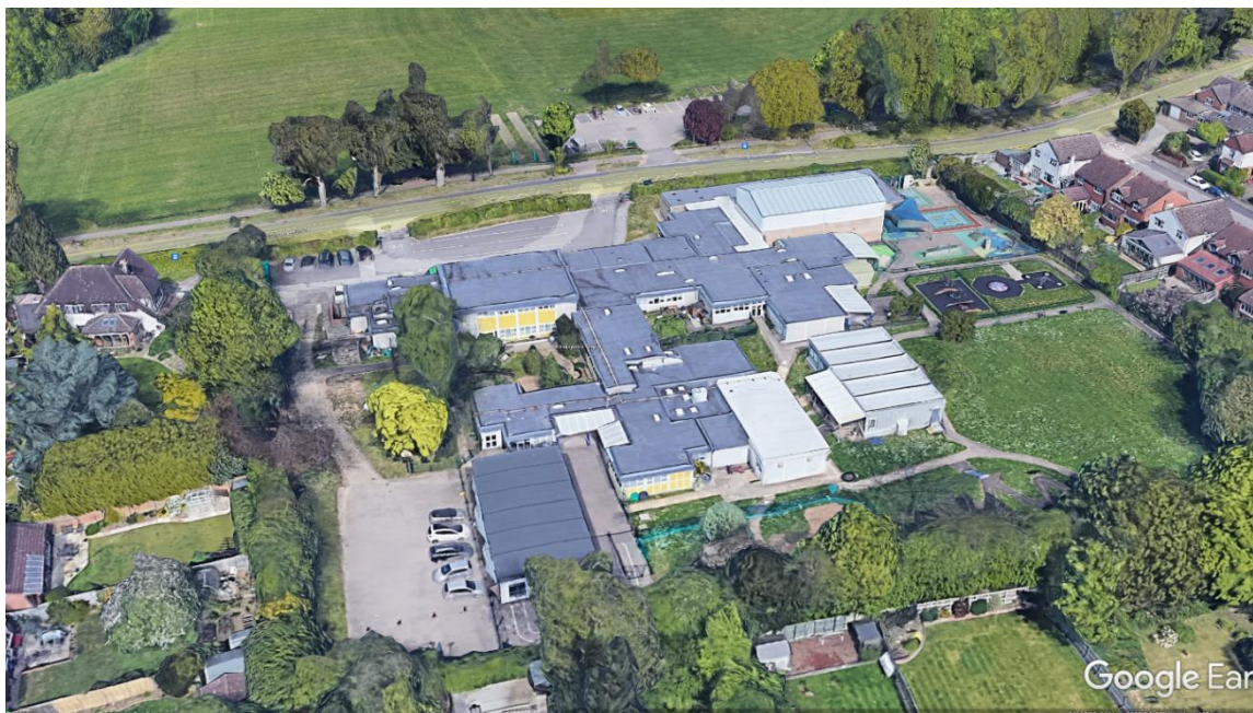
Aerial view of Breakspeare School, Abbots Langley (Copyright: Google Earth)
