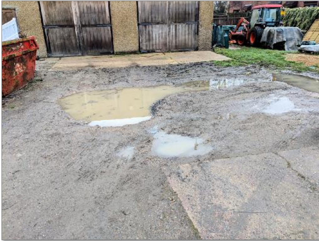
Depot Surface (Images taken 05/02/2019)
